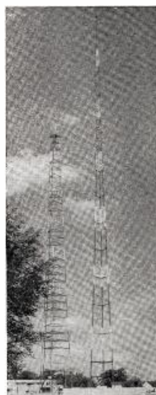
WKBN-TV Truscon Self-Supporting Tower 539-Feet Tall
