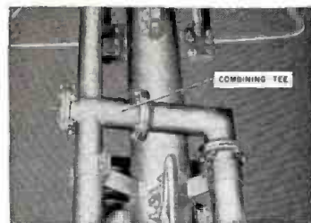
TEE FEED divides power proportionately between upper and lower bay groups.
